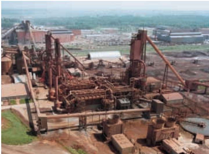
DR-Plant with briquetting of fines with binder
