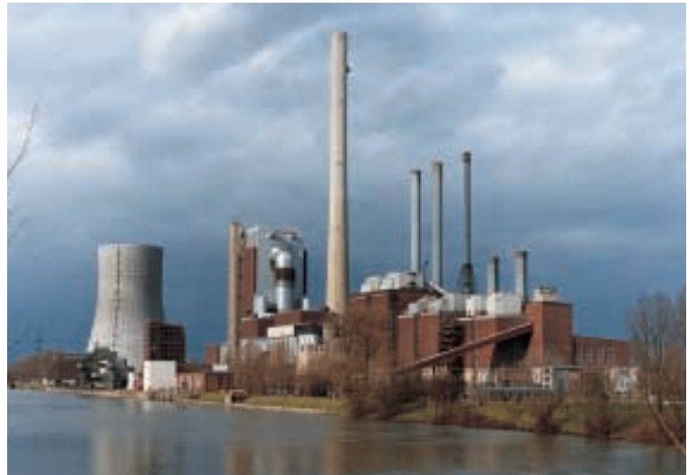
Coal-fired power plant with FGD and binderless gypsum briquetting units
